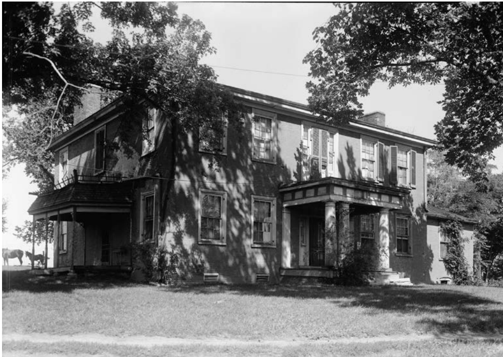
Capt. W. D. Swinney’s Glasgow residence, Sylvan Villa, built about 1845. Image courtesy of Historic American Buildings Survey (HABS)
