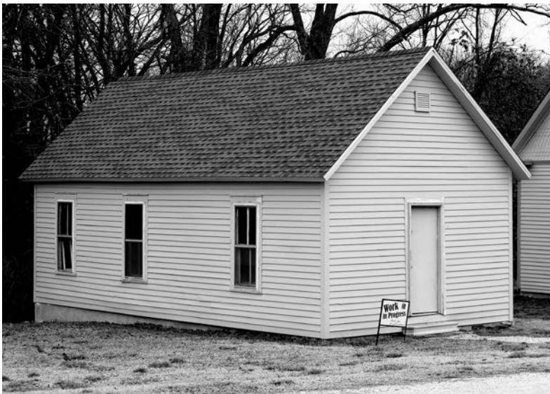
The partially restored McQuitty shotgun house which is now located on the grounds of the Boone County Historical Society Museum.
