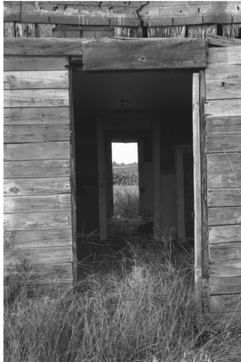
THROUGH THE SHOTGUN —Abandoned shotgun house clearly shows the logic of the above term, where doors from front to back were aligned. Photo by Brett Rogers
