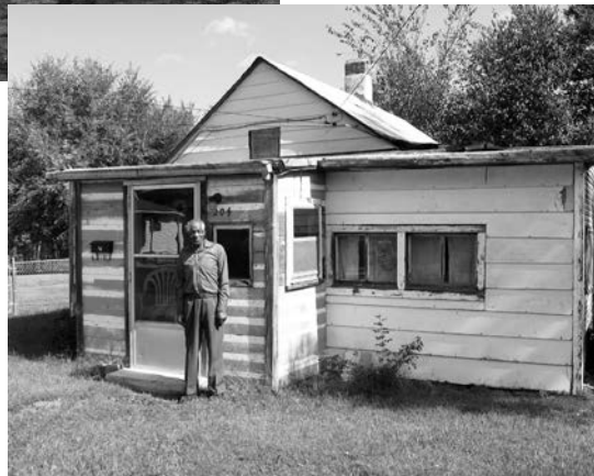
Top: Side view of the Lewis Patrick shotgun house shows the successive additions made to the back and side of the house over the years. Lower: Lewis Patrick in front of his Louisiana Drive shotgun house in 2007. The house was later damaged by a fire and then torn down in 2012. Patrick died in 2011.
