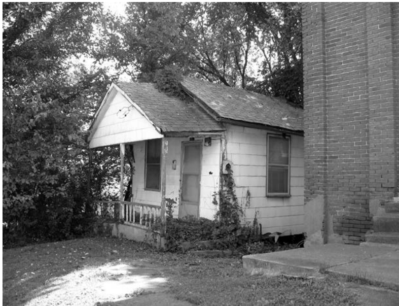
Before it was torn down several years ago, the Enyard family's 500-square-foot shotgun house stood next to Campbell Chapel AME Church in Glasgow. A five-room house, it was a rare example of the shotgun style. The first two rooms were bedrooms and it had a small basement kitchen. The house had not been lived in for some time.
